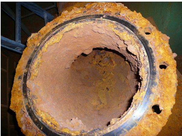
**Fig. 1: Cast iron pipe with manganese containing deposit in a drinking water pipe**
